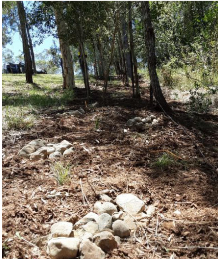
After installation of rocks and planting, 25/11/22
